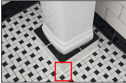
3.0 Item 6(Picture) Example/ Sample- Second level Hall Bathroom
