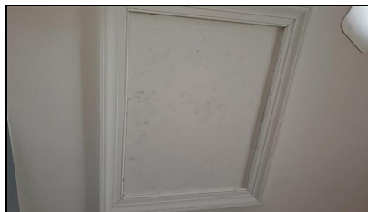
8.0 Item 3(Picture) Example/ Sample- attic access panel(s)
