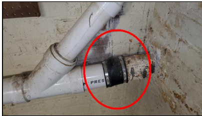
5.3 Item 2(Picture) Example/ Sample- Example/Sample- floor joist – deteriorated/damaged wood member(s)
