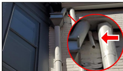
7.5 Item 1(Picture) Right side of home-
