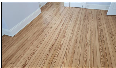
3.0 Item 1(Picture) Example/ Sample- Second level Rear Bedroom
