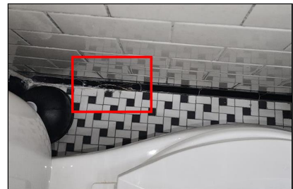
3.0 Item 5(Picture) Example/ Sample- Second level Hall Bathroom
