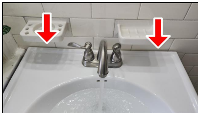
3.0 Item 11(Picture) Example/ Sample- Second level Hall Bathroom
