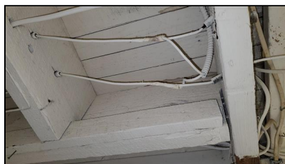
6.4 Item 4(Picture) Example/ Sample- basement
