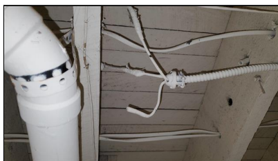
6.4 Item 5(Picture) Example/ Sample- basement
