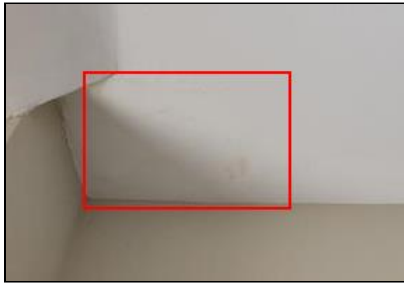
3.0 Item 2(Picture) Example/ Sample- Third level Front Bedroom
