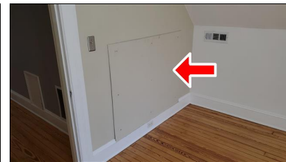
8.0 Item 2(Picture) Example/ Sample- attic access panel(s)
